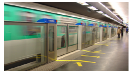
Kaba Gilgen AG's Platform Screen Door Systems in Paris Metro Station
